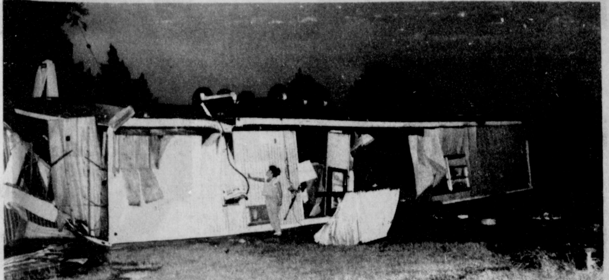
HIGH WINDS AT WAKA overturned this mobile home owned by E. O. Drake. Other wind damage was reported throughout this community as well as in Hansford county in and around Gruver.
