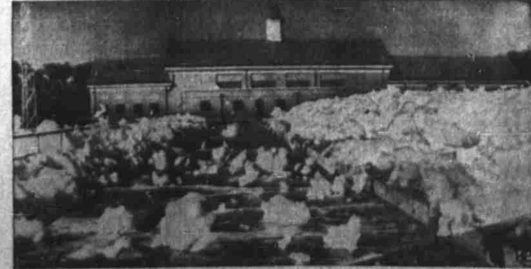
IT'S NOT SNOW —These banks of "snow" are suds foaming up from aerating basin at sewage disposal plant in Knoxville, Va. Plant's manager said large amounts of detergents in sewage being treated combined with oxygen in churning water to create the suds.
