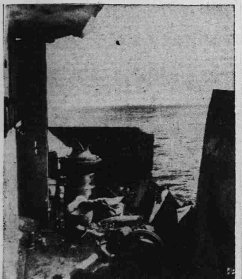
WRECKED BRIDGE OF U.S.S. NEW MEXICO—The port side of the battleship U.S.S. New Mexico's bridge looked like this after being hit by a Japanese bomb in Lingayen Gulf Jan. 6, 1945, while supporting American landing on Luzon...
