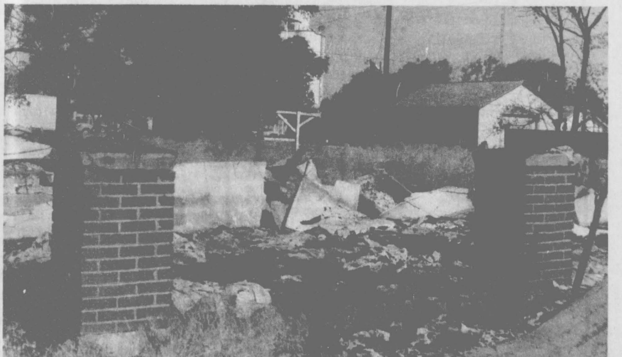
This is what is left of what was a broken down house on the corner of First and Barkley Streets. The Spearman Volunteer Fire Department burned the structure to the ground last Monday night. They
