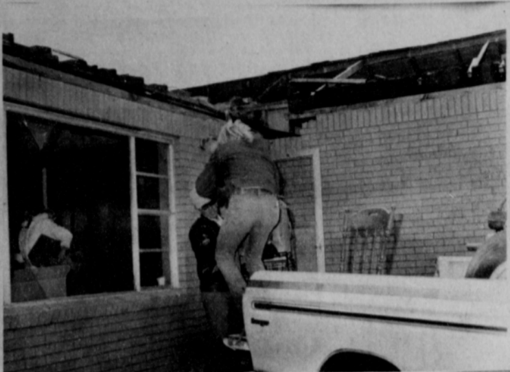
This is front view of the Dennis George home, which was struck by a tornado Wed. 4 a. m.
