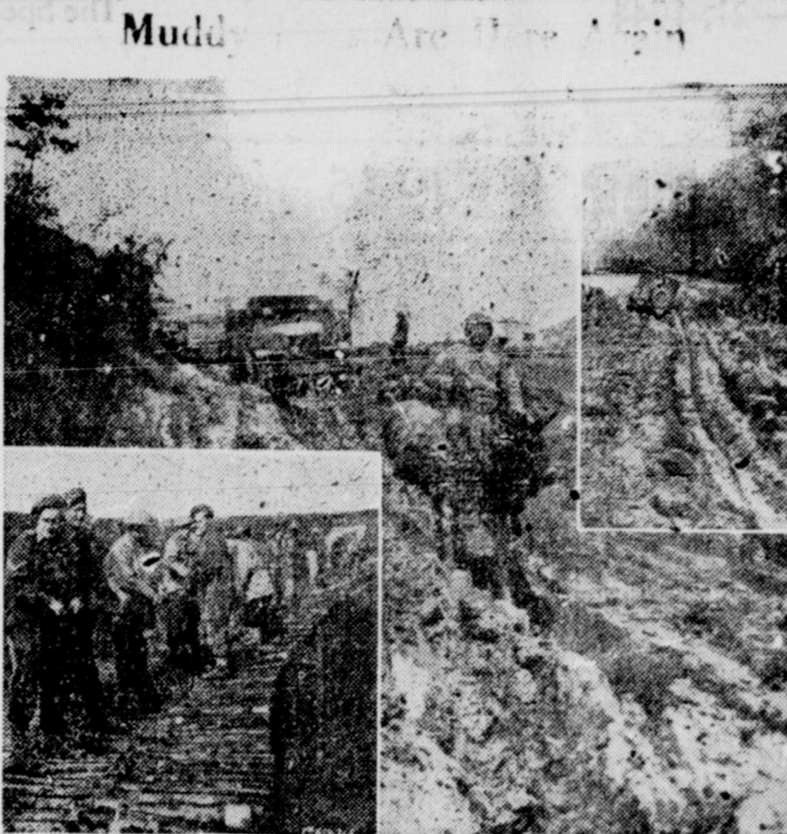
South African troops in Italy have built this road (lower left), out of 105-mm. shell cases, in order to pull their 40-mm. Eofors over it for the Fifth army. Center—Mules are used to carry supplies south of Bologna when the mud gets knee-deep. Upper right—Hub-deep with mud, the Italian roads have slowed down supplies. In many sections it is necessary to fly in almost all material on account of impassable roads. Thousands of miles of roads are now being constructed by American engineers in France and Italy. While the construction takes time, many of the new roads are in operation.
