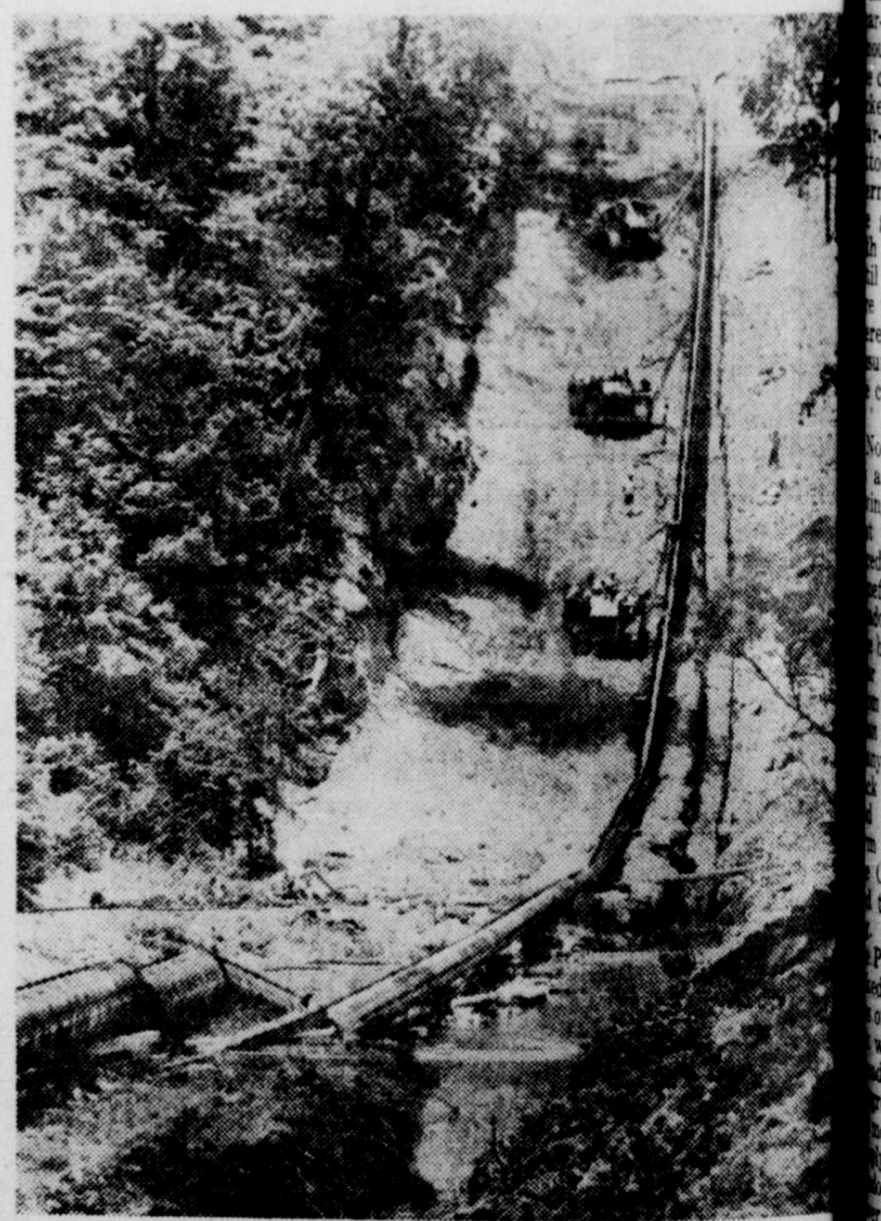
Laying the Big Inch pipe line across Allegheny mountains in Pennsylvania.
