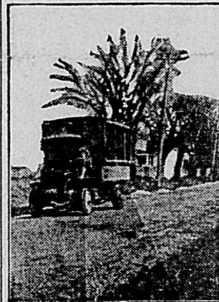
Overloaded Truck Increases Danger of Cutting Surface of Improved Roads.
