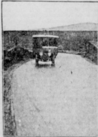
Hard Surface Road Built by Federal and State Funds.
