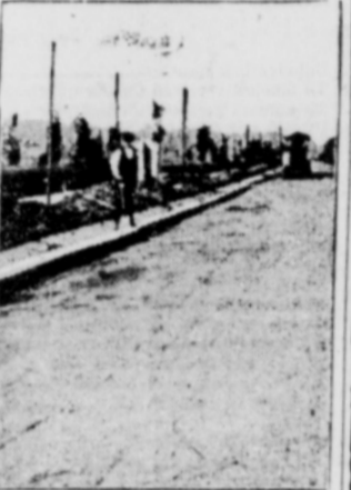
Construction of Concrete Road.
