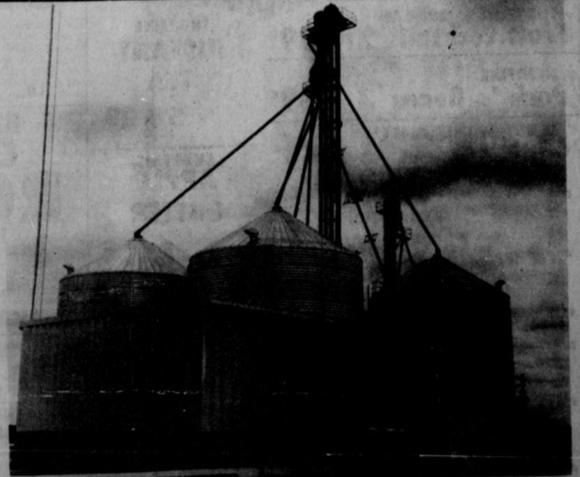
Pictured above is the beautiful new 4-Tex Elevator located south of Spearman. The beautiful new facility presently has a 284,000 bushel capacity. The directors of 4-Tex announced this week that the elevator will be increased by 254,000 bushels to make a total of 540,000 bushels, in time for the corn harvest. Directors include Charles West, George Jackson, Dr. Earl Novak, and Pat Patterson.
