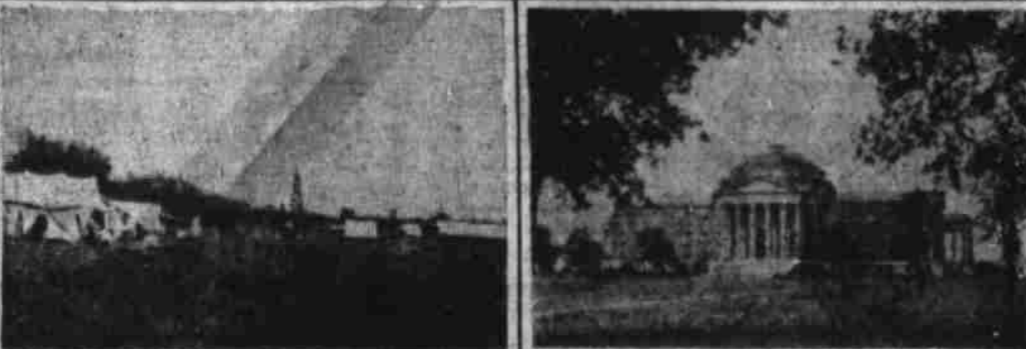
S. M. U. CAMPUS, 1914 CAMP FOR CONSTRUCTION OF DALLAS HALL
