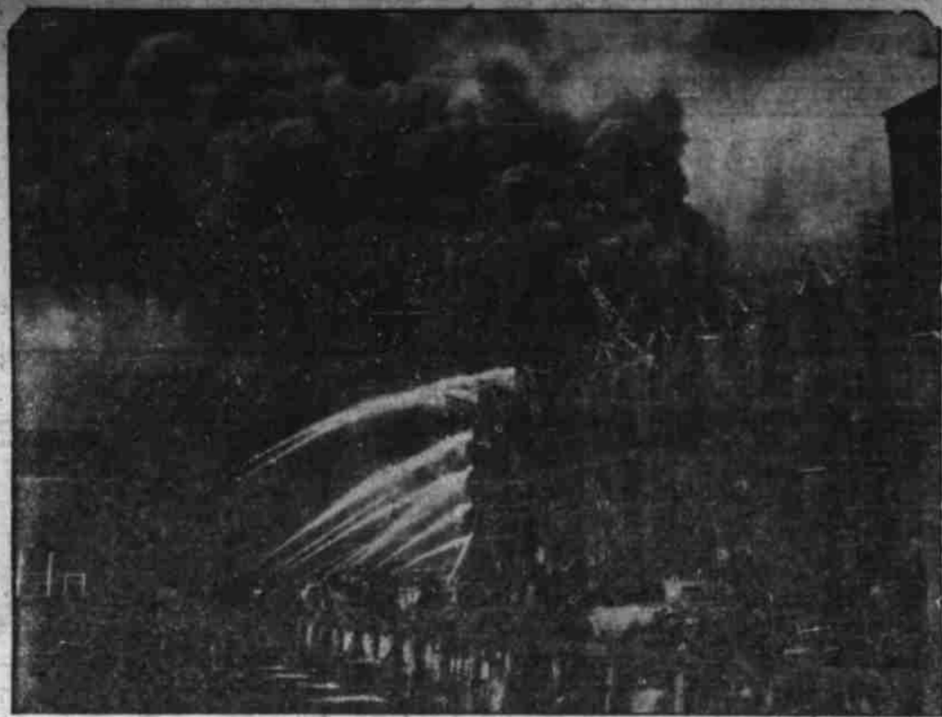
Rolling forth great clouds of smoke to cast a pall over Brooklyn and Manhattan, a five-alarm fire swept an immense warehouse on the Brooklyn waterfront. This spectacular photograph was made while the fire was at its height. More than 50 firemen and other persons were injured or overcom. (Associated Press Photo)
