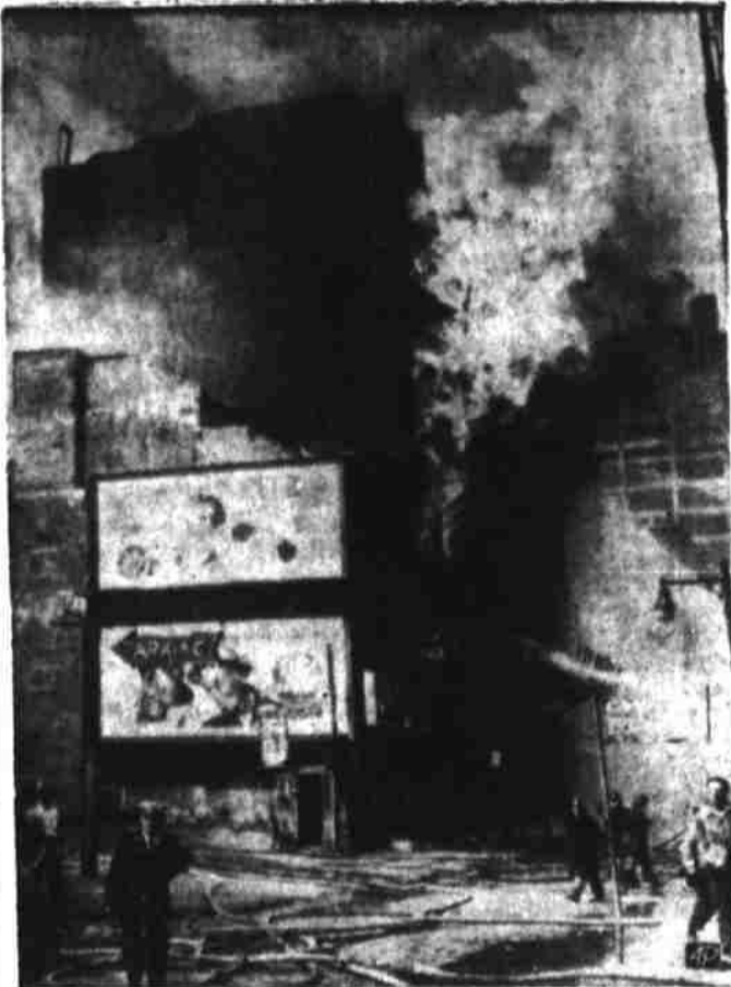
FOUR ALARM FIRE SWEEPS WRECKED BUILDING —Flames pour from a vacant building on Philadelphia's downtown Sansom street as four alarms sent 40 fire trucks to the scene. The building, fire officials said, was being dismantled when the blaze started. Several nearby buildings were set afire but these fires were quickly extinguished. Cause of the blaze was not determined. (AP Wirephoto).
