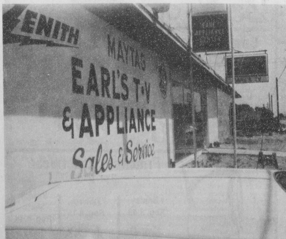
LOCAL FIRM EXPANDS -- Construction of an addition to the building occupied by Earl's TV and Appliance is now underway. The move marks a growth by the city of Spearman to this point and the faith of the owners of this firm in the future growth of the city and its businesses.
