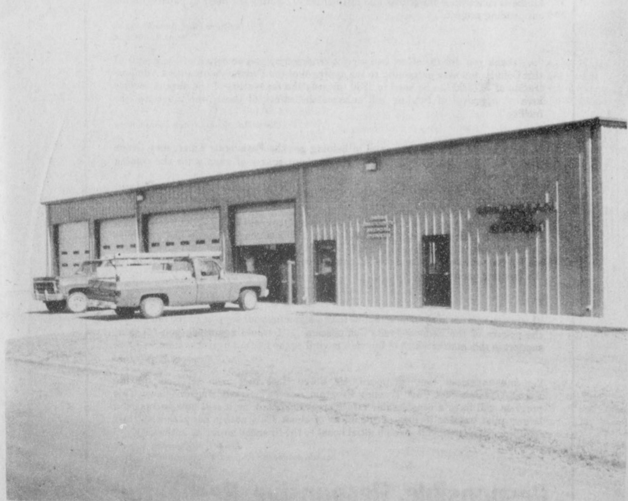
NEW FIREFIGHTING HEADQUARTERS -- A part of the pact to finance and build a new fire station was for the volunteer firefighters -- they volunteered for this, too -- to do interior completion work themselves. This they have been doing in addition to their regular jobs and firefighting duties. Helping them are Roscoe Nelson supervising work on the building; John Trimmell, plumbing; Lawrence Anthony, electrical work and Clay Gibner, finances in the form of a loan.
