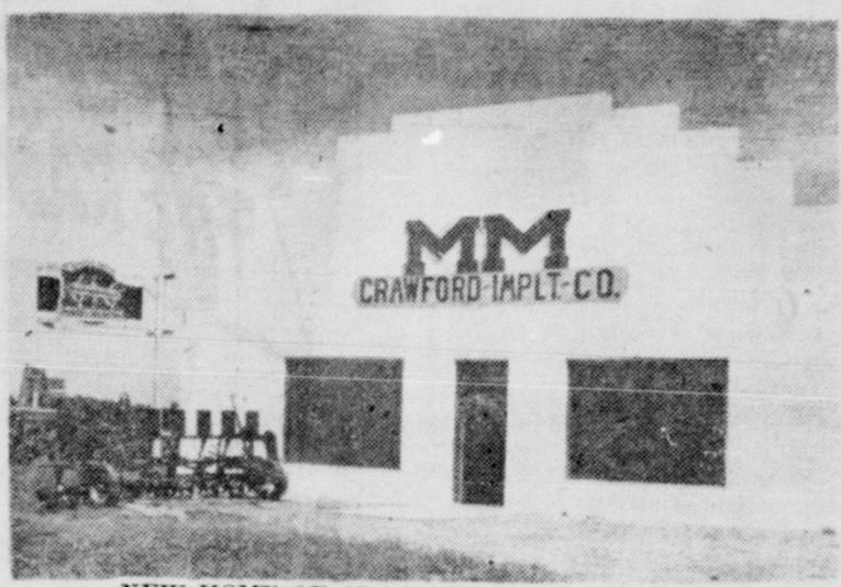
New Home of Crawford Implement Co.
