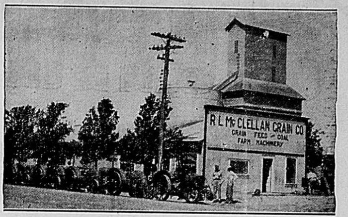
The earth was broken this week to run the foundation for an annex to the R. L. McClellan Elevator. There will be five new units of storage increasing its capacity 35,000 bushels. Every caution is being made to insure safer storage, The weather will gauge the time of construction—so says the voice of experience.
