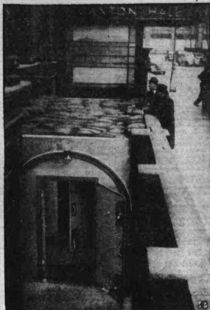
AIR-LOCKS TO KEEP OUT GAS and splinter-proof steel doors feature London's newest air-raid shelter.
