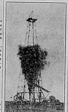
Picture snapped just a few seconds after 290 quarts of Nitro had been set-off in a Shell-Sinclair gas well on the W. L. Russell farm in Moore county. The well was treated with two 5,000 gallon treatments of acid the next few flays after the "shot" and finally registered a railroad commission registered a railroad commission registered a railroad commission second soon cubic feet of
