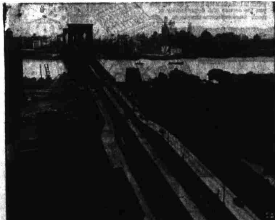
KEEPING AN OLD LANDMARK GOING — View of famed Brooklyn Bridge from lower Manhattan, N. Y., shows extensive repair work being done on approaches and structure.
