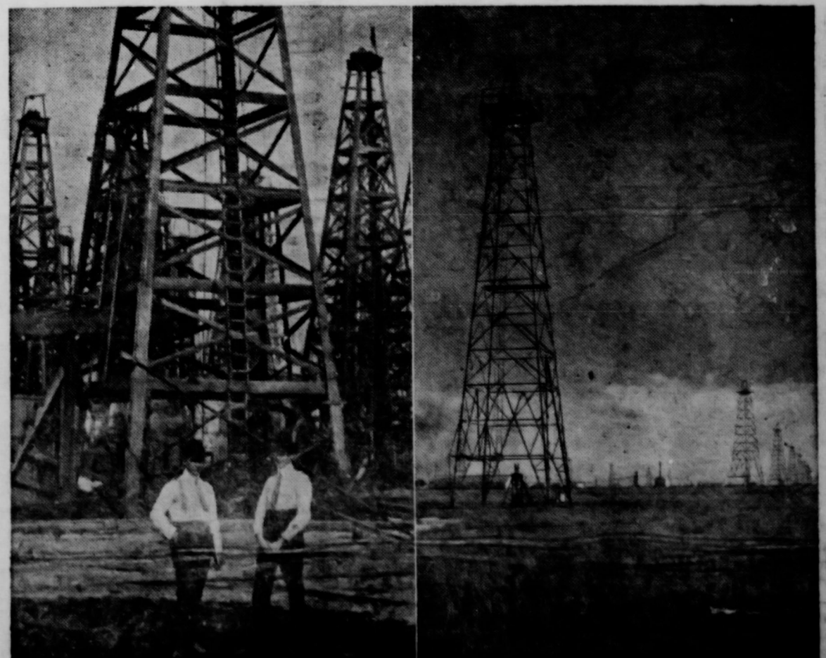
PROGRESS IN CONSERVATION is clearly illustrated by these two photos from Humble files. At left are wooden derricks of a generation ago, closely spaced for quick - though wasteful - production, as outmoded as the fashions of the men pictured. At right is a modern oil field in the Panhandle, with steel derricks marching in a scientifically
