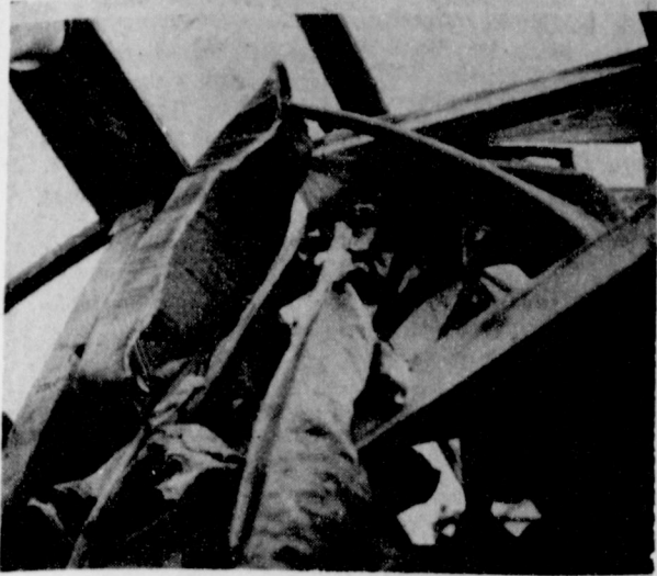
It is not an airplane wreck, but a banana tree pushing through the roof of the greenhouse at Robert Novaks in Spearman area!
