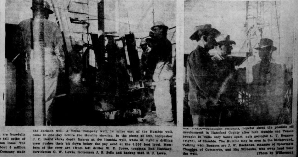
HANSFORD COUNTY GAS GAMMER - Residents of Spearman are hopefully seeing the horizon open miles northwest of this city where the tall spike of a drilling rig cuts into the sky on the S. P. and K. K. Jackson lease. The well blew in several days ago with a driftest test showing about 6 million cubic feet of gas mixed with distillate, Humble Oil and Refining Company made the Jackson well. A Texas Company well, 10 miles east of the Humble well, came in one day before the Humble shooting. In the photo at left, topusher J. C. Beard checks depth figures at the Humble well, while at right a drilling crew pushes their bit down below the pay sand at the 5,000 foot level. Members of the crew are (from left) Driller W. D. Jones, tongman Bob Hubbard, derrickman G. W. Lewis, motorman J. B. Sells and backup man E. J. Love.
