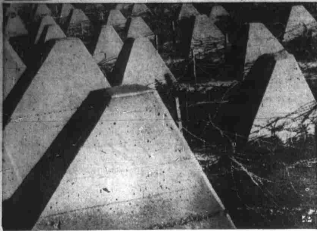
NO THANKS FOR TANKS —With military activity along the western front stalemated by weather and by the apparent respect each high army command has for its enemy's fortifications, German sources distribute this picture of their concrete tank traps, designed "to protect the German frontier from sudden attacks." Note barbed wire interlacings.
