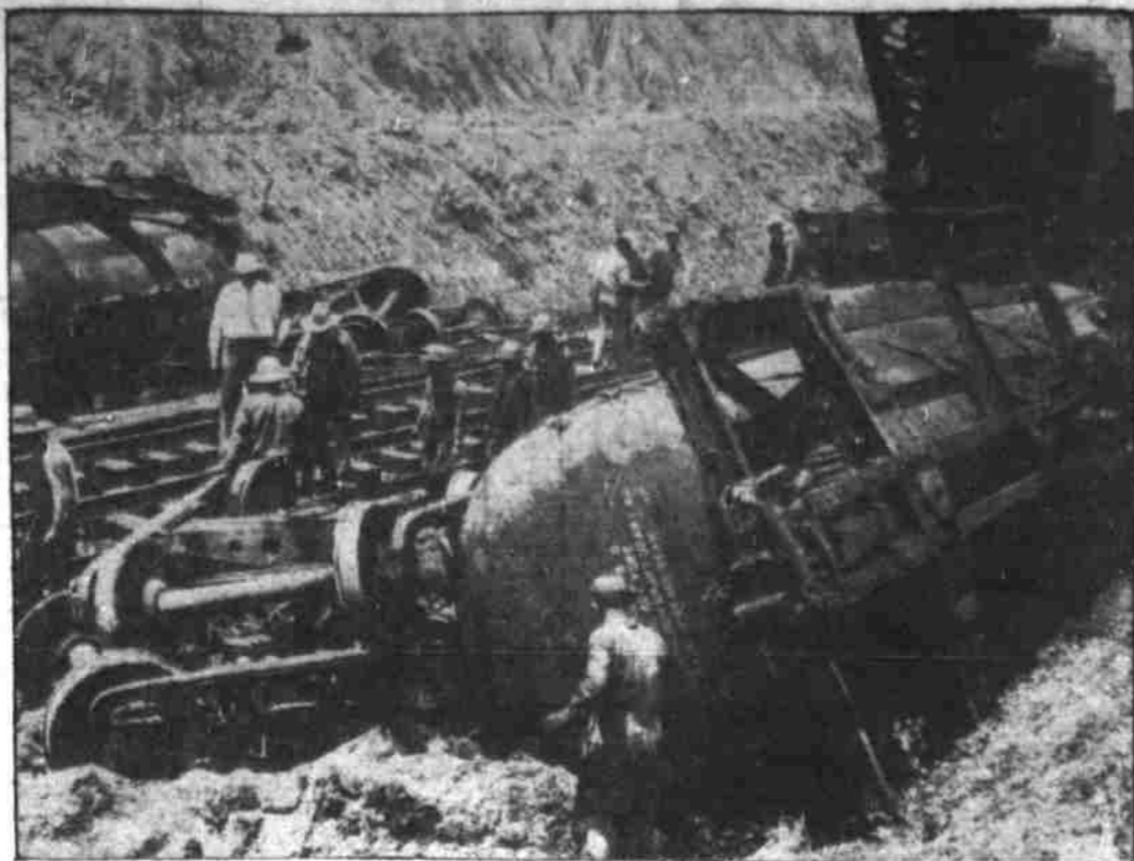
Crews working feverishly Thursday morning to clear the Texas and Pacific tracks of wreckage after freight cars derailed east of Coahoma. A Herald photographer snapped a view of the twisted cars a short time after the wreck occurred.
