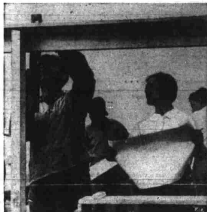
DOING THEIR SHARE. women worked alongside the men in building a new Jewish settlement at Mirfaz, Palestine. Inside of two days, the settlers converted a swampland into a camp complete with watch-tower, enclosure and huts.
