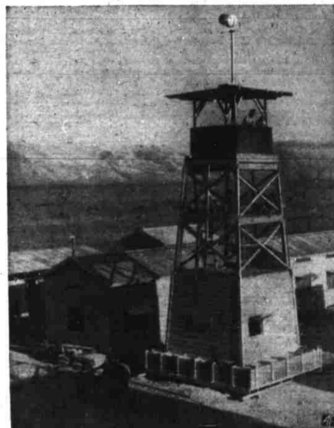
DAWN-TO-DAWN LABOR of Jewish colonists replaced a Holy Land swamp with a new refugee settlement at Mirfaz, and even the above watch tower was put up by the feverishly-hurrying builders. Settlers buy their land on leasehold terms, with payments spread over several years.
