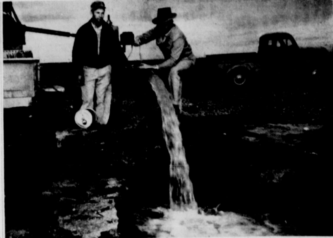
LIQUID TREASURE in the form of irrigation water is shown in the above photo made recently on the John Belaska farm one mile east of Glenn, just inside the Dickens county boundary. Mr. Belaska (left) and S. J. Braselton, Jr. are making a "draw-down and orifice test on the hole." The well was drilled by Wade (Mutt) Beryman of Matador and developed by Braselton Implement Company of Roaring Springs. Flow is 320 gallons per minute from the 109-foot well, sufficient to irrigate about 60 acres of cotton under the sprinkler system. Irrigation is spreading rapidly in the area below the Cap Rock. An irrigation school is announced for February 22 at the Spring Theatre. Roaring Springs, conducted by an A. & M. Extension Service. The program begins at 9 a. m. all farmers in Motley and Dickens counties interested in irrigation are urged to attend. Problems of financing, development, water sources, etc. will be discussed.
