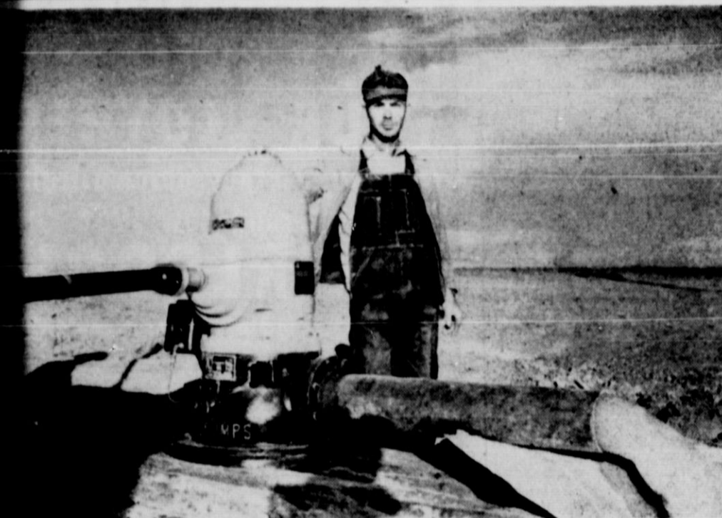
ANOTHER PRODUCER in Motley county is the 500 gpm irrigation well shown above on the Avery Payne farm about five miles east of Roaring Springs. Mr. Payne (standing beside pump) says he believes that irrigation is the answer to most of the problems faced by the farmer. The well, drilled by Milt Berryman of Matador and developed by Braselton Implement Company of Roaring Springs, is 150 feet deep and it is estimated to irrigate 100 acres under sprinkler system. An irrigation school is being conducted next week (Wednesday, February 22) at the Spring Theatre, Roaring Springs. An irrigation expert from A&M Extension Service will conduct the program starting at 9:00 a. m. "Tuition" is free.
