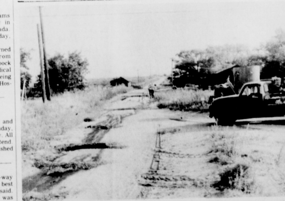
OIL ON THE ROAD — This scene shows oil on a road near the Jack Luckett home at the northeast corner of the town section. The oil on the surface resulted from a leak in the Scurlock Oil Company's (of Houston) line July 20. The leak was under the Northfield Farm To Market highway. Small dams were built to prevent the oil from running into fields. It was later sucked up into a large truck. The line carried oil from the Roaring Springs fields to Whiteflat, about 20 miles.
