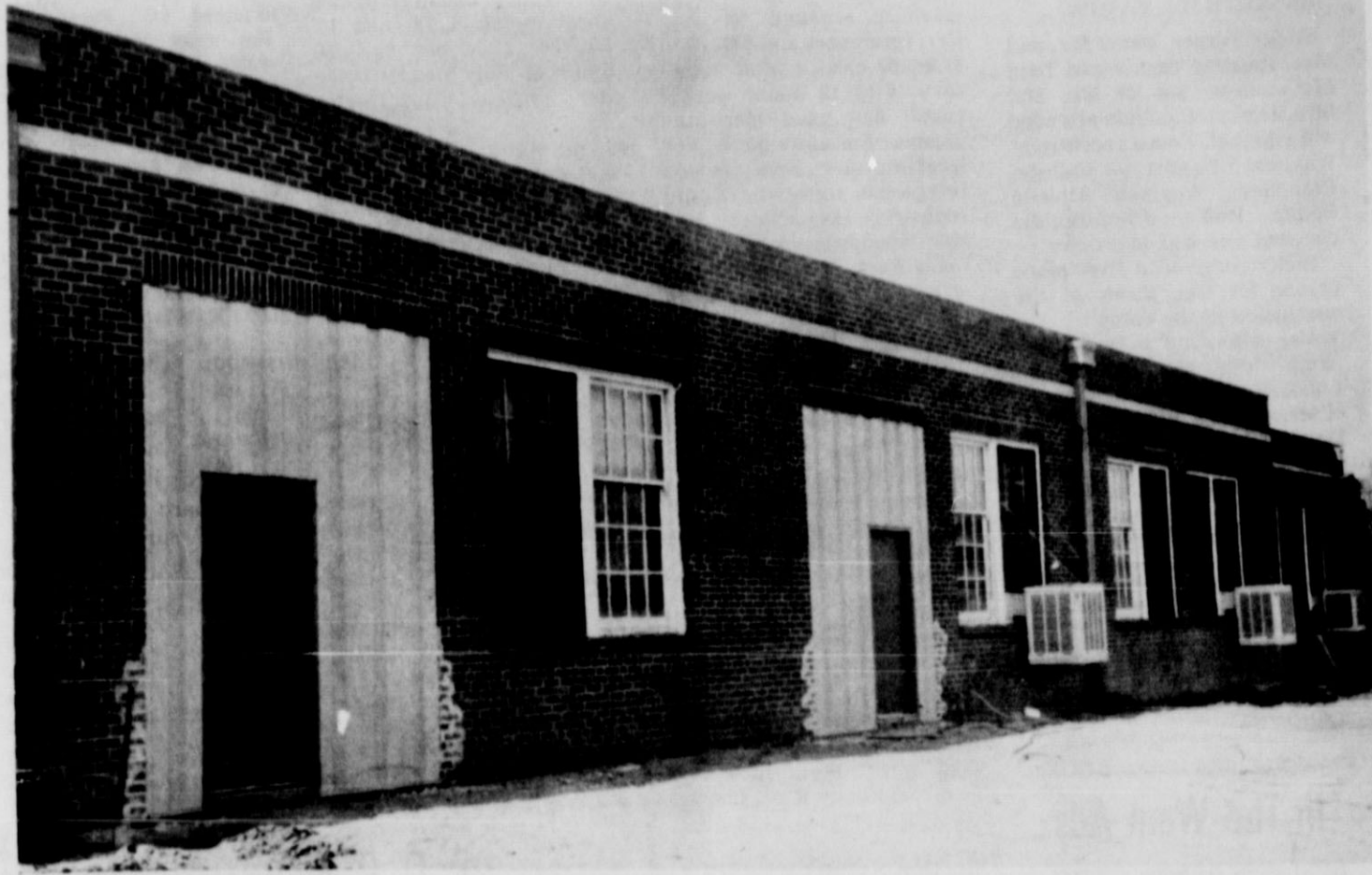
NEW DOORS on the former grade school building which will house the agriculture department when the building program is completed. These doors are on the south side of the grade school building but will be on the inside of a new shop addition, now
