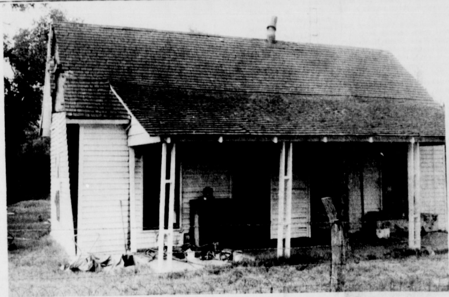
HISTORIC old Mott line camp house on the Burleson Ranch. Photo shows the west gable dislodged by the explosion as was the east end of the old building. William Ratze was severely
