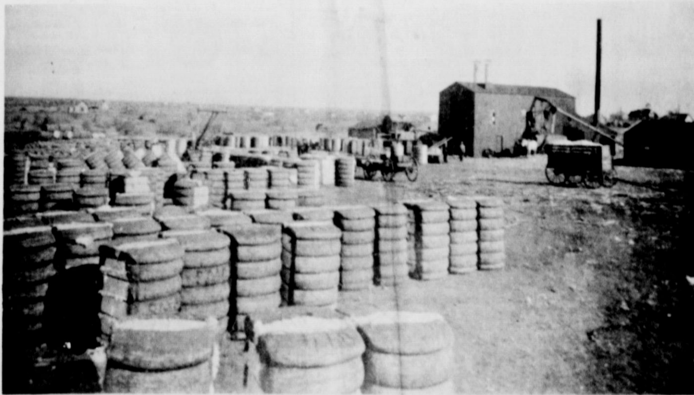
THIS is the first gin in Matador and was owned by T. G. Duncan (a native Scotchman) and Jack Luckett, early pioneer and businessman. The photograph was made about 1901. The plant was located in southwest Matador, and was rebuilt in 1912. In 1918 it was sold to West Texas Gin Company, and moved to Meadow, Texas in 1920.
