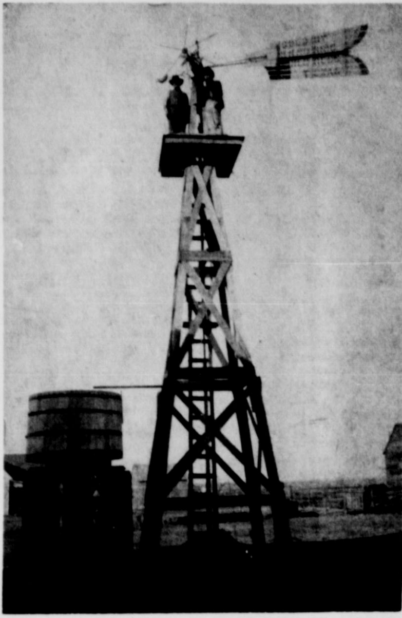
EARLY WATER SYSTEM - The Tribune has no information on the above photograph, except that the two men are identified as Dick Wheeler and Bob Meador. Lettering on the vane of the mill says "Sold by R. H. Norris, Childress, Texas." Parts of the wheel are on the ground, indicating that mill is new and being put into operation. At one time information declared the mill to be on the northwest corner of the courthouse square, but it can not be confirmed. —Source of photo unknown
