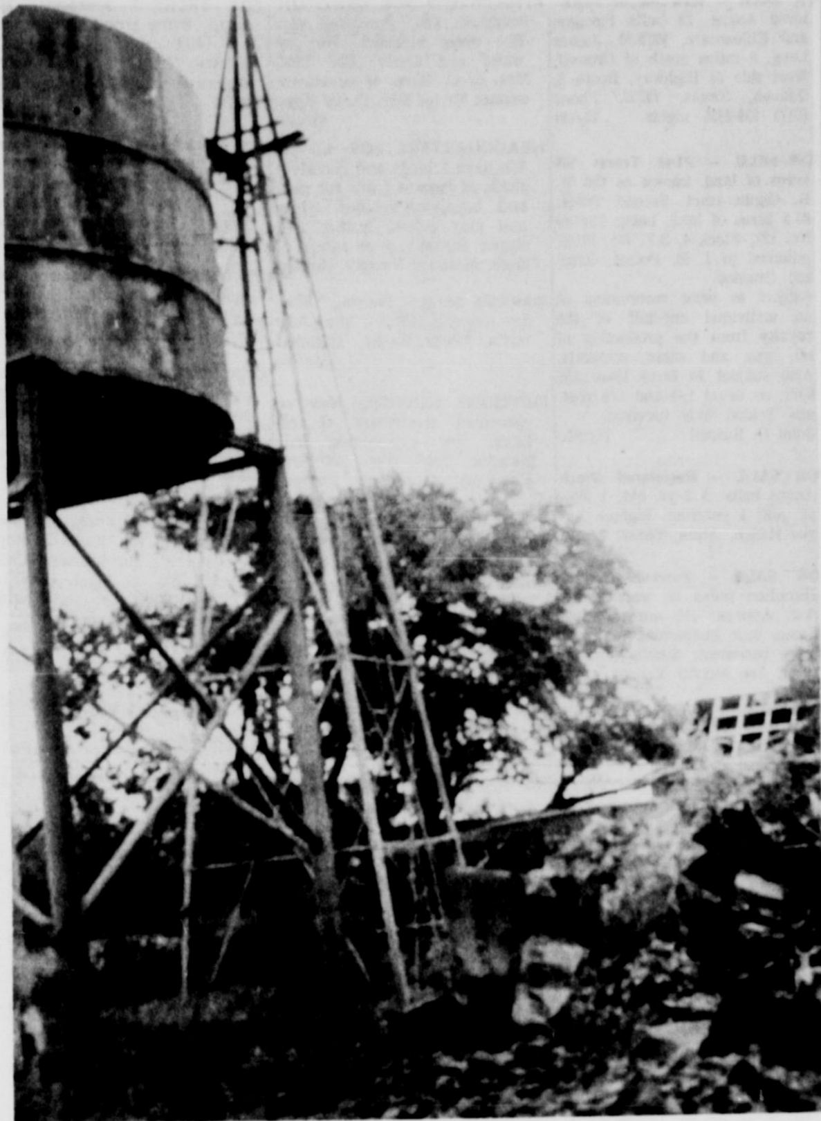
ANOTHER WINDMILL that fell during the storm that lashed this area late Thursday. It was on the former Walter Carpenter farm, operated by E. A. Day. The wheel shown at the lower right, was hanging about midway on the tower after the storm passed. Part of the unroofed barn is shown in background. — Tribune photo
