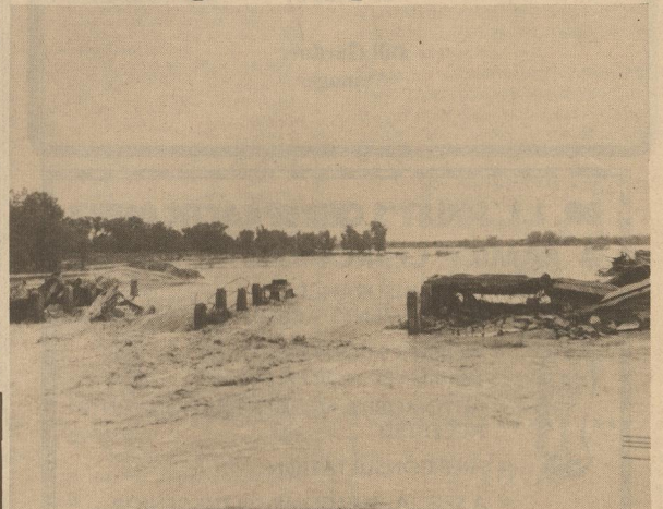
In this picture you can see the tremendous amount of water that swept through the bridge which collapsed. This is the old bridge.
