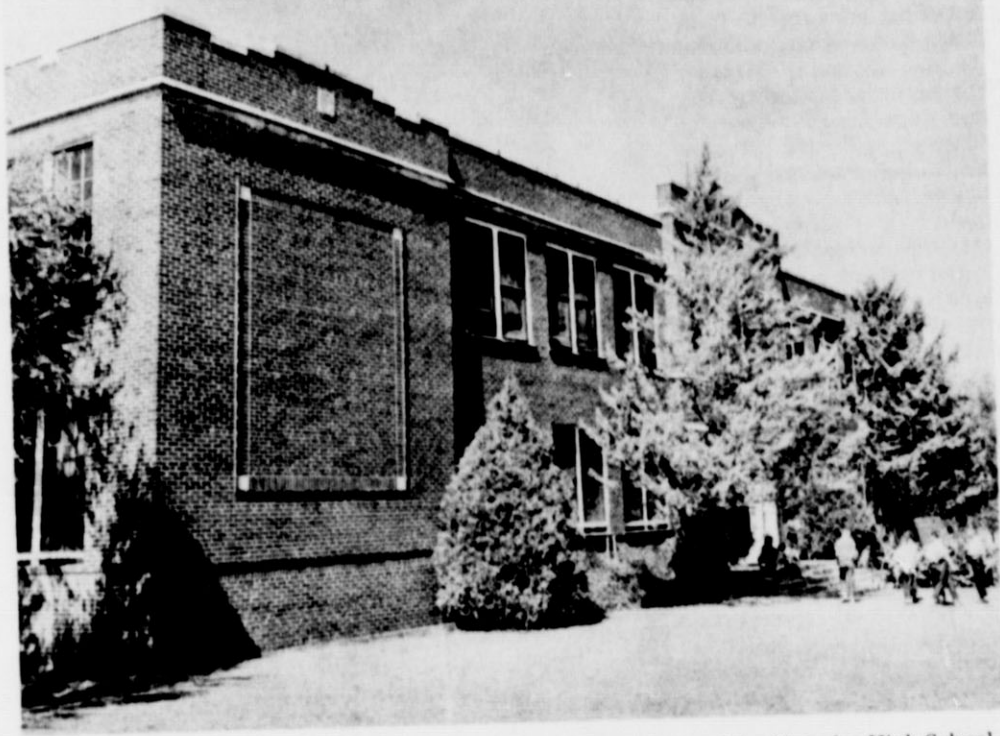
BUILT in 1925, many graduates have passed through the doors of the Matador High School. The last class, however received diplomas from the auditorium stage Monday night. Disposal of the structure has not been announced by the Motley County Independent School District board of trustees.
