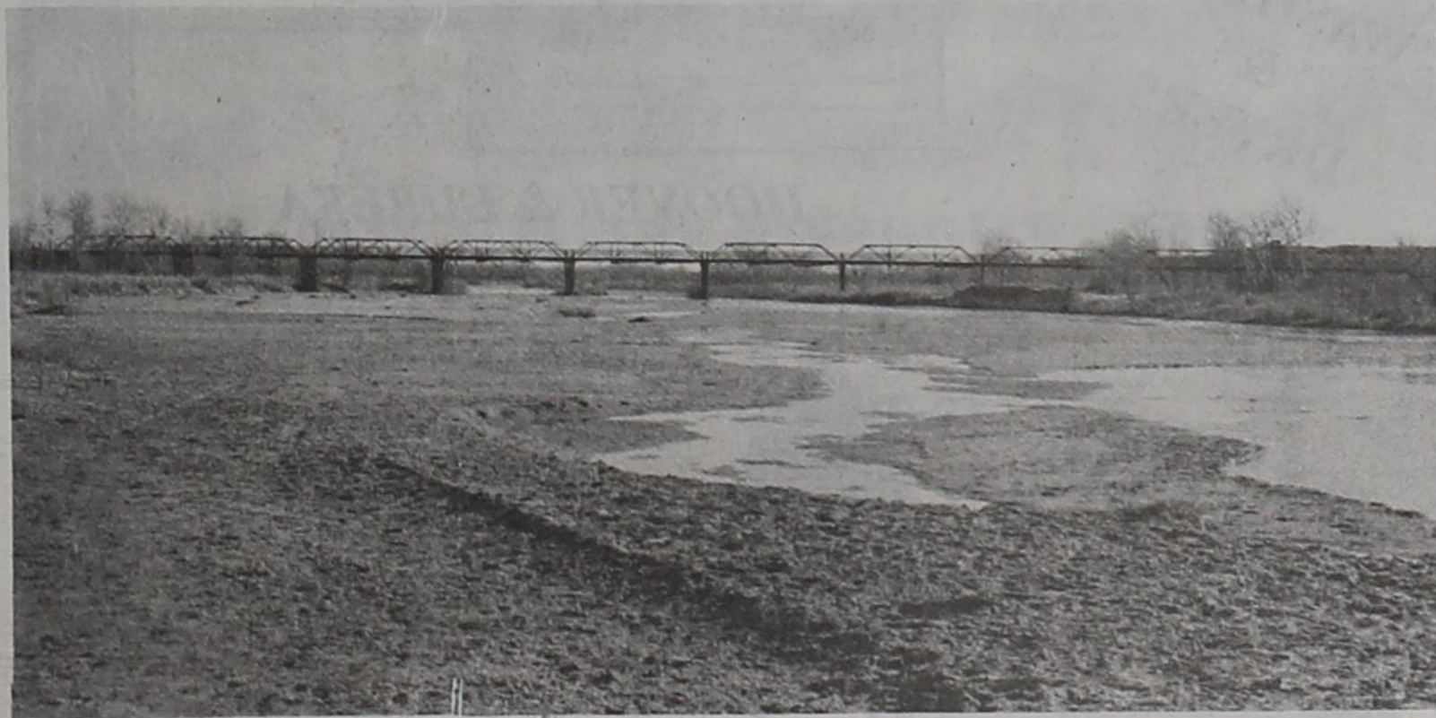
DUMONT BRIDGE — This long county bridge located near Dumont will soon be rebuilt. The bridge is approximately 450 ft. long, but will be shortened some when refurbished.
