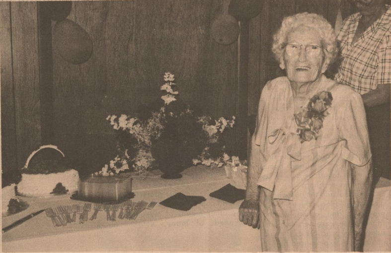
Minnie Van Bridge
