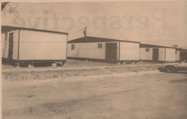
PORTABLE CLASSROOMS- Four portable classrooms were moved onto the Motley County School campus last week. The buildings will house grades four, five and six and Special Education/Title I Reading. (Photo by Mary Renfro)
