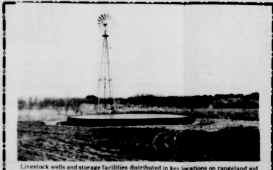
Livestock wells and storage facilities distributed in key locations on rangeland aid in better range management.
