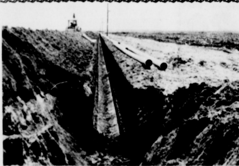
Underground irrigation pipeline conserves water through more efficient use.
