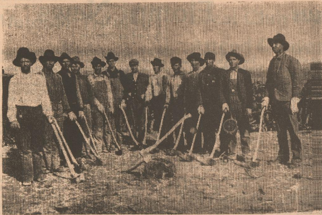
A PLACE TO BUILD A CITY — These workmen were clearing the land to build Roaring Springs in 1913. The names of five are known, reading from left to right, No. 3 is Walter Carpenter, No. 4 is Jim Swaringen, No. 7, is Nelson Pender and No. 12 is Oscar Callaway. This photo courtesy of Brooks Callaway.
