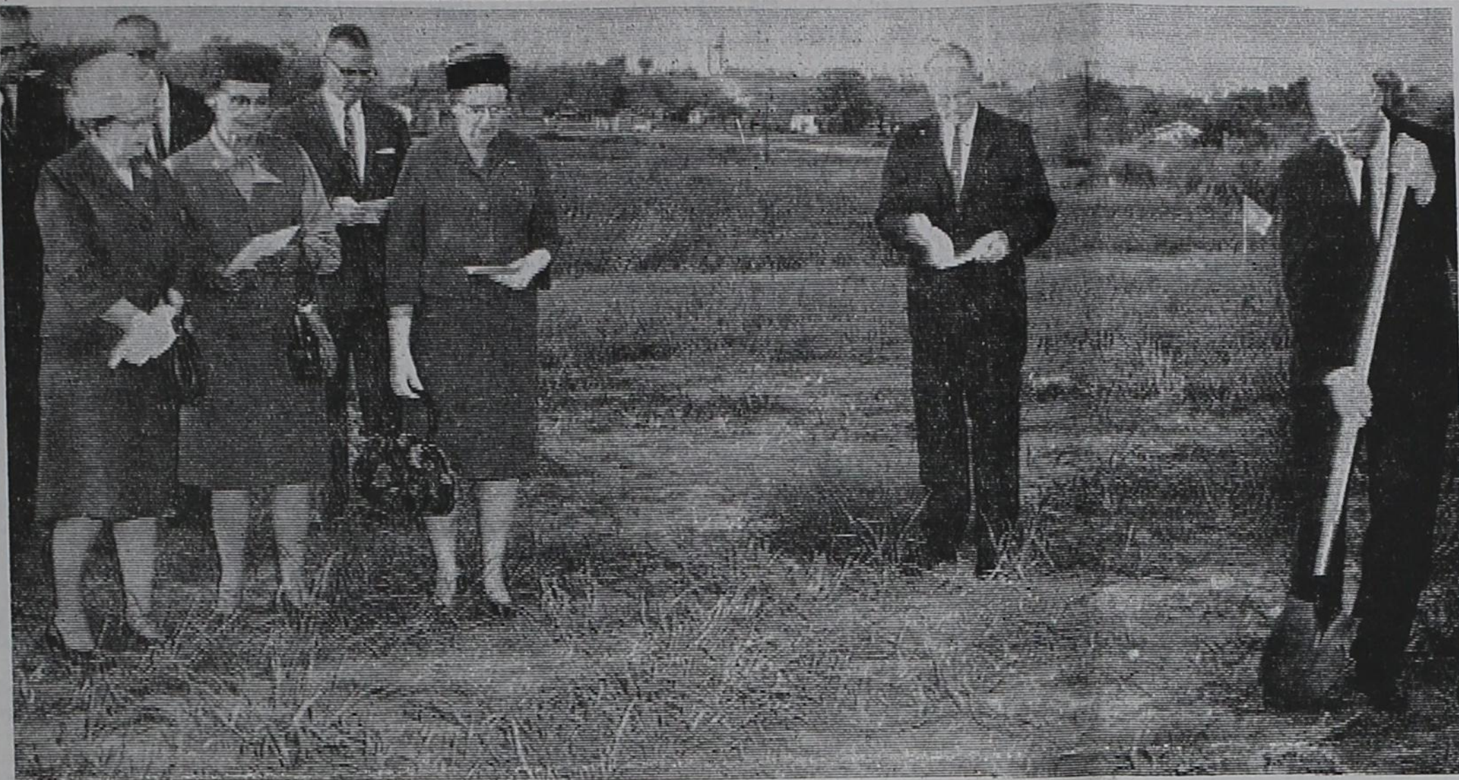
GROUND BREAKING CEREMONY, held November 14, 1965 by the Roaring Springs First Baptist Church, for a new church structure, was the fulfillment of a lifelong dream by the members. Participating were members of the Women's Missionary Society, the Board of Deacons, and church and Sunday School officers. Shown in the above picture from left are, back row: M.S. Thacker, Charles Long and Buck Pruitt. Women are, from left, Mrs. Lem Miller, Mrs. M.S. Thacker, and Mrs. T.B. Yeates. Rev. C.A. Butler, pastor, is shown at center, and at right is J.P. Cooper.
