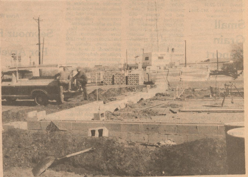
The building of new Allsup's store in Matador.
