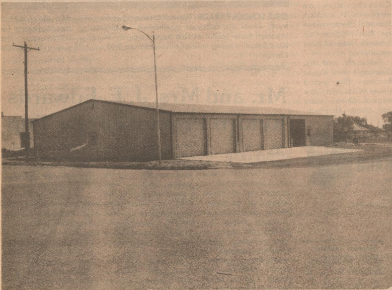
NEW FIRE HALL - The Matador Volunteer Fire Department officially moved into its new headquarters May 24 on the east side of the courthouse square. (Photo by Leon Watson)
