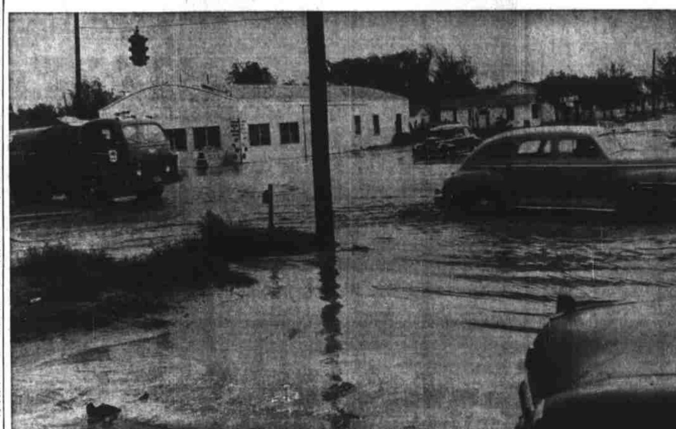
Downpour Floods City Streets Water covers the intersection of West Third and San Jacinto Streets, slowing traffic to a crawl following a brief but intense shower early Thursday afternoon. Water also raced down streets in the business district, flowing curb to curb in some spots, as approximately one inch of rain fell within half an hour. More rainfall during the night boosted the total for the 24-hour period to 2.22, according to measurements at the U. S. Weather Bureau at Webb AFB. (Staff photo by Keith McMillin).
