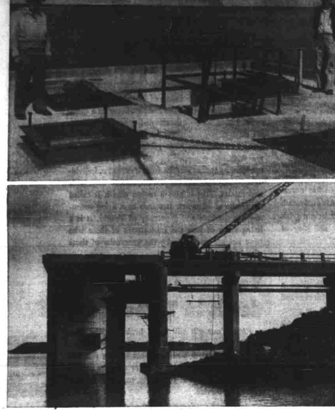
Ready For The Pumps
