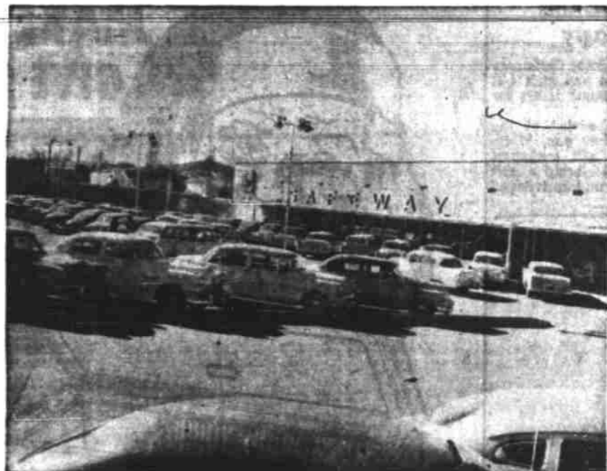
This scene shows the parking area of the new Safeway on opening day. Even though there's free parking for 192 cars, the lot was filled to capacity all day long. As soon as cars moved off, there were others waiting to move in.
