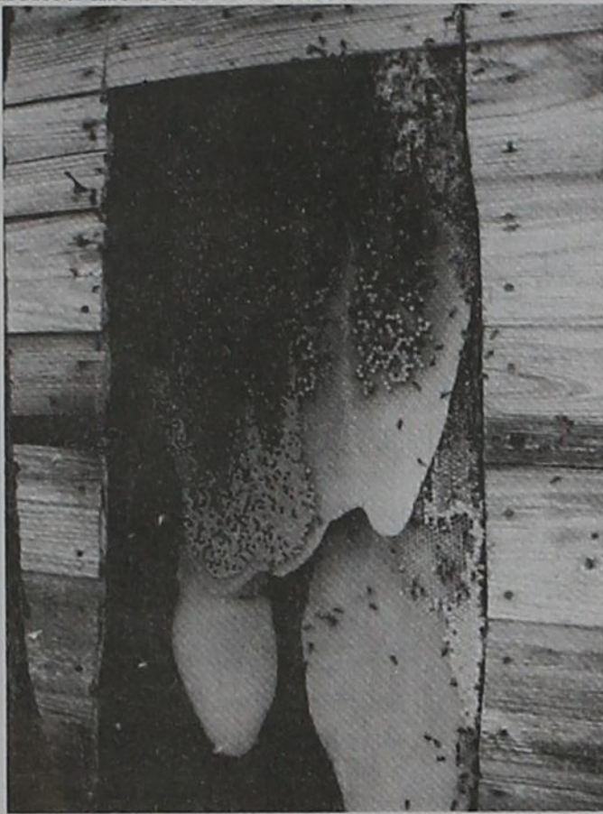
The picture shows the lay-ers of comb in the hive. The picture shows about six verti-cal feet of comb. In this struc-ture, the bees built three dif-ferent layers of comb. Most
