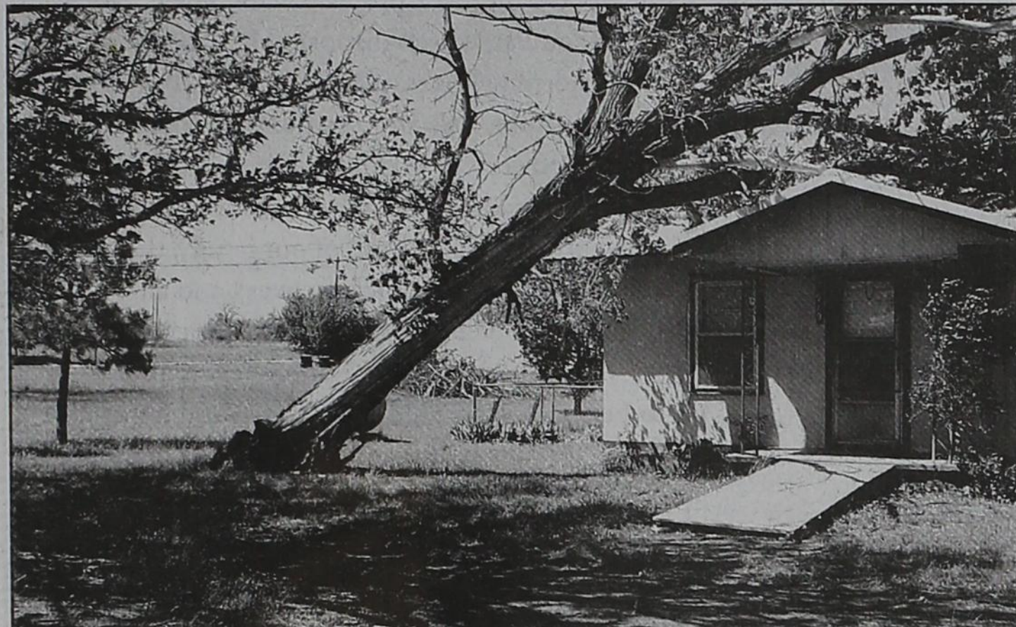
Wind blew a 55 year old cottonwood onto a house with a new metal roof. The two month old roof sustained a minimum amount of damage. The house is occupied by Bessie J. Williams who was unhurt. She said she had her hearing aids out and still hear all the noise. The West Texas mesonet registered 55 mph winds this past Friday.
