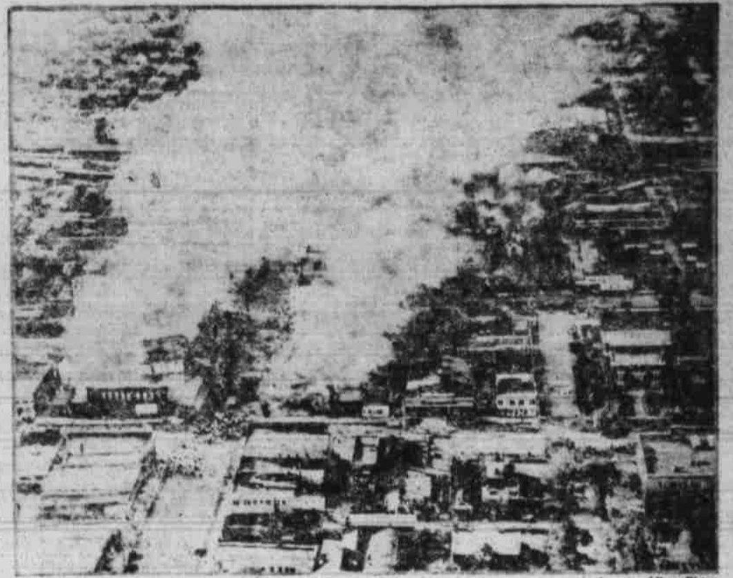
This air view shows the $2,000,000 fire at Spencer, Iowa, in which 30 buildings in the business district were destroyed. Explosion of fireworks in a drug store window started the conflagration.
