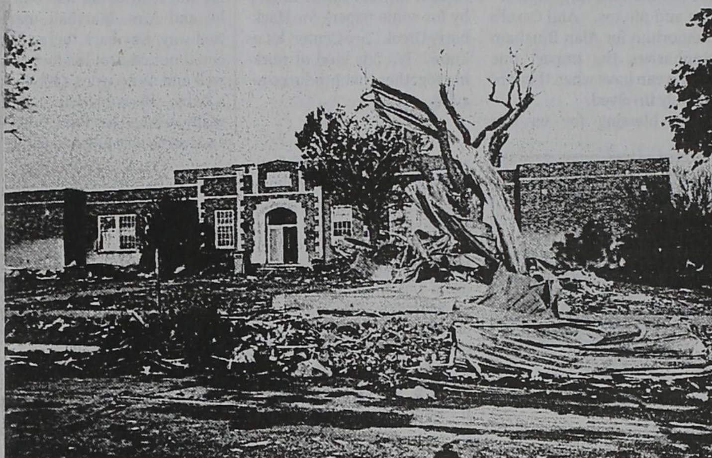
Debris litters the lawn of the old elementary school, a block southwest of the school. The Matador Elementary, still standing, and built in 1930, survived a direct hit. (Photo courtesy of Billy and Brenda Osborn).
