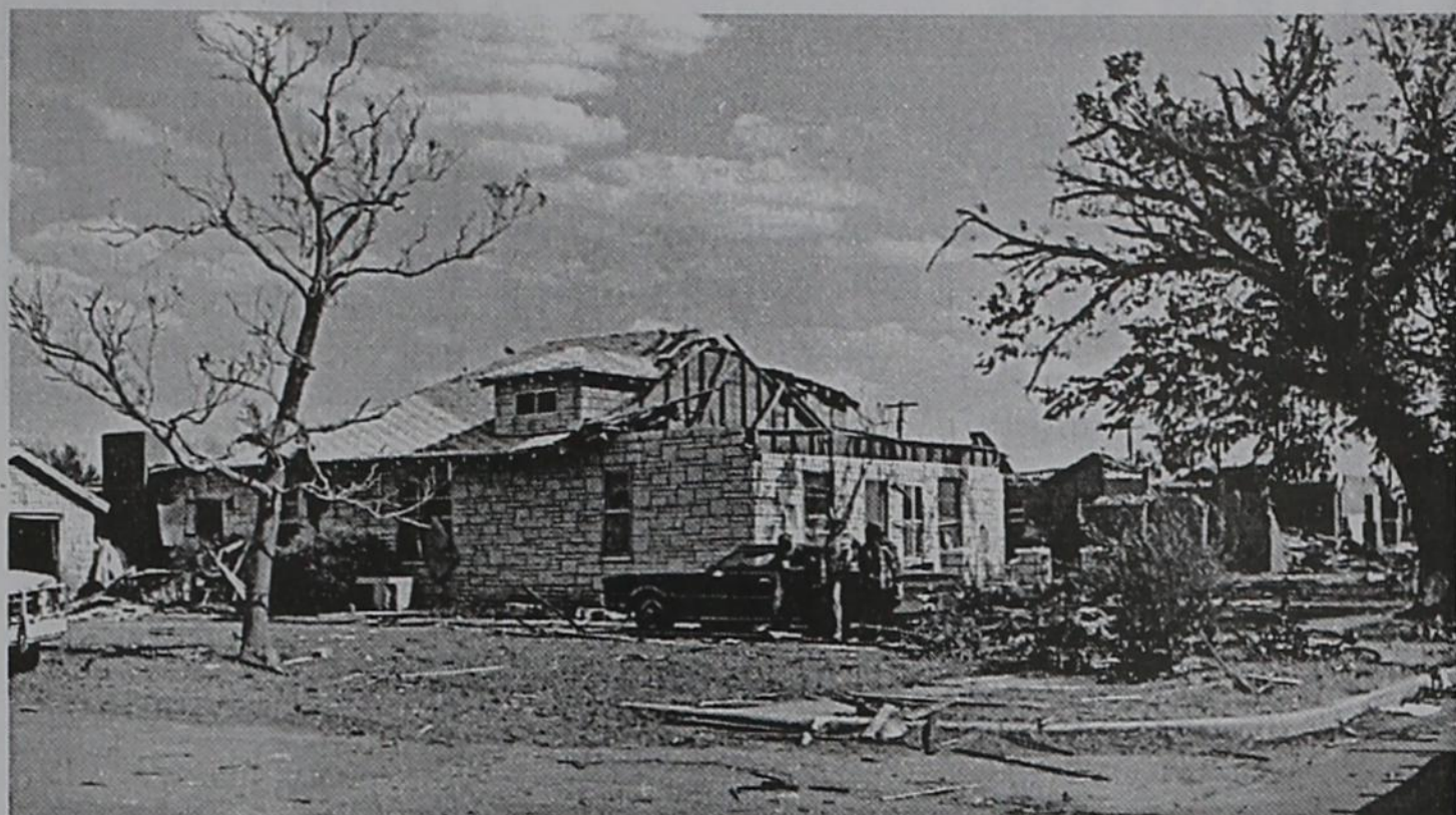
The morning after, surveying the damage - the roof was gone on the front of the house, and not visible, to the east, a tree destroyed the rear den and kitchen. An interesting note: Gerald's baby grand piano survived the implosion, but when he raised the key cover, a 2-by-4, "as if someone had cut it to fit," Gerald said, was lying on the keys.
