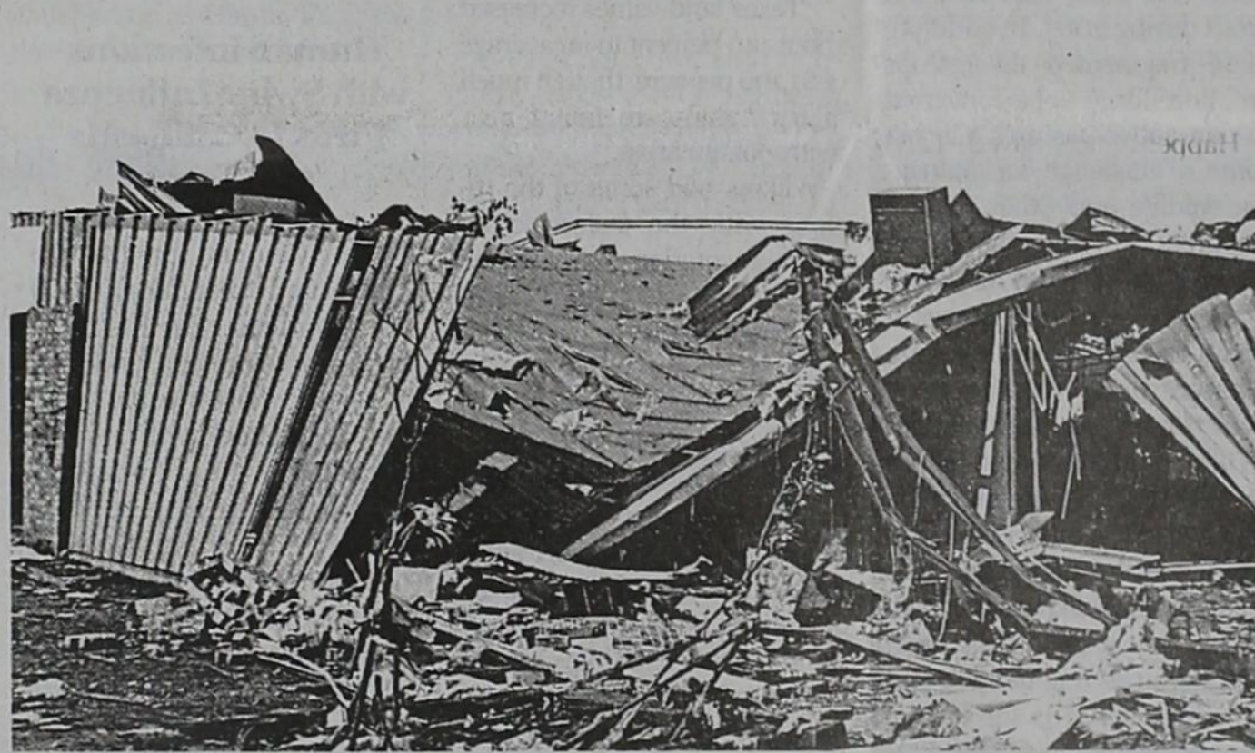
The grade school was totally destroyed. This photo shows the damage to the southwest corner. (Photo courtesy of the MC Athletic Booster Club).
