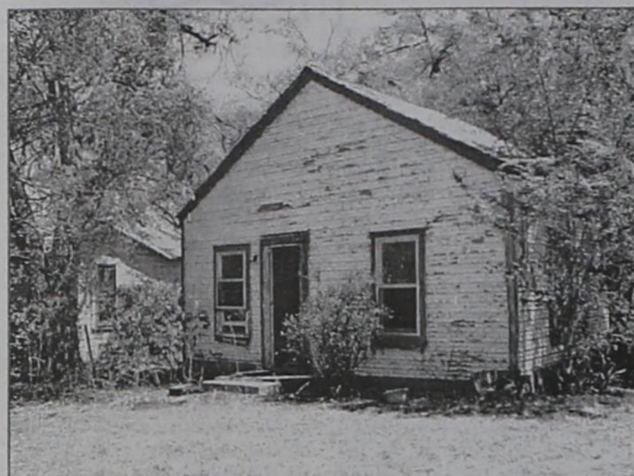
SUBSTANDARD DWELLING in first block of Second Street in Roaring Springs scheduled to be demolished.
