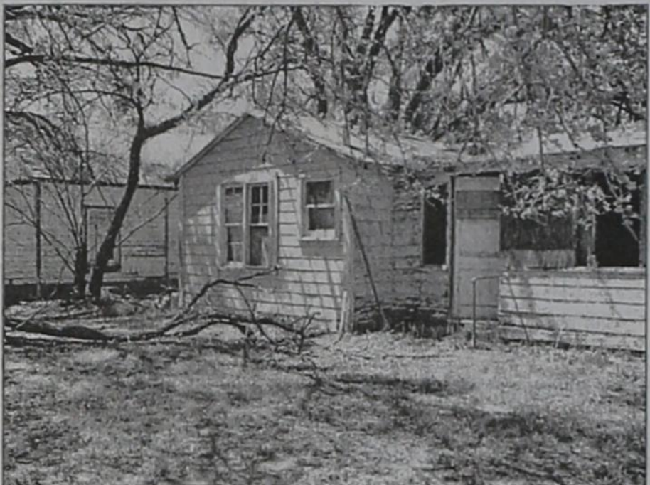
SUBSTANDARD DWELLING on corner of Second Street across from US Post Office in Roaring Springs scheduled to be demolished.
