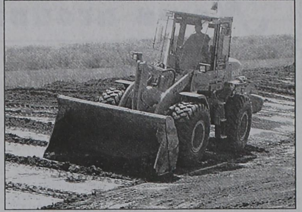
Motley County TxDOT employees work to prepare roads for winter weather.
